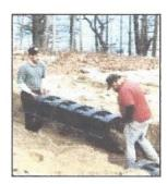
Leaching chambers are successfully replacing gravel and pipe for leach field installations. Their lightweight construction allow for easy hands-on installation with minimal soil compaction. The product is adaptable to serial and lateral projects. Today, leaching chambers have grown in acceptance and total 30% of leaching systems installed.
