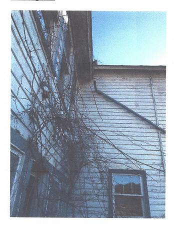
S&A recommends that all of the downspouts present at the perimeter of the home be repaired and attached to non-perforated drainpipes and extend/daylight approximately 15 feet from the foundations.
