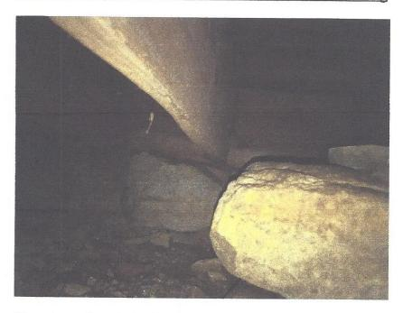
The primary foundation for the Main House consists of stone masonry. Generally, the foundation appears to be in overall good condition and does not appear to be in need of immediate repairs. At various locations, masonry repointing efforts have been completed.
