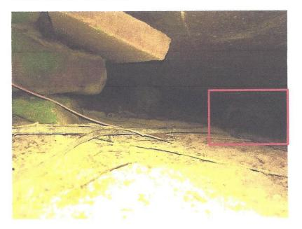
At one location within the crawlspace, a single CMU pier is present. The pier at this location is likely in need of reinforcement. However, this is a relatively minor repair that your brick/stone mason can rebuild without additional guidance from our firm. However, when you get to this, please feel free to contact me, and I will be happy to provide a specification for this pier reinforcement.
