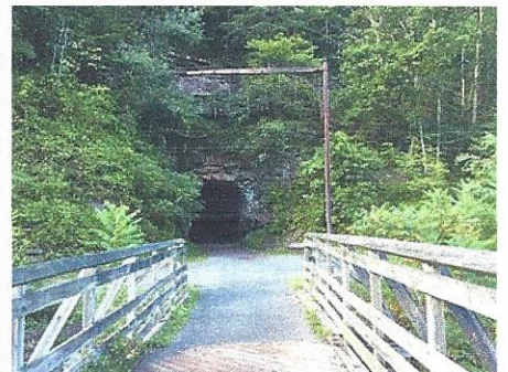
Southern entrance to Sharps Tunnel
