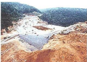
Gathright Dam construction
